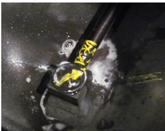
Leak location at welded joint between the nozzle and the nitrogen line
