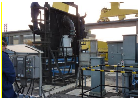
Electric driven auxiliary pumps for low Danube water level
